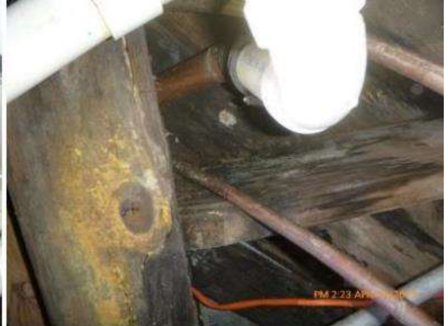
Sagging or dipping was observed. Unlevel flooring observed. Multiple Locations. Broken Structural members observed. Example kitchen floor.
