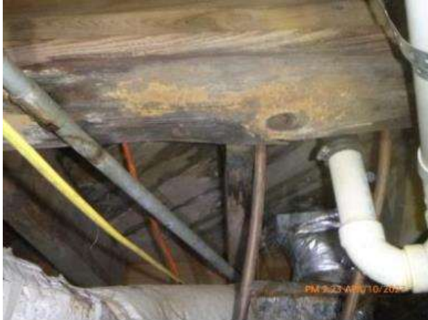
Sagging or dipping was observed. Unlevel flooring observed. Multiple Locations. Broken Structural members observed. Example kitchen floor.
